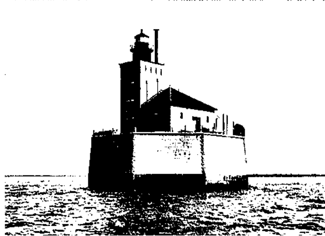
Notice steam whistles and quoining on brick-faced crib
